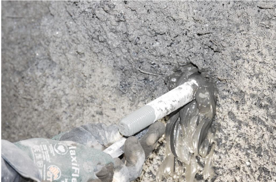
Figure 27. Removal of protective tape from bolt.
