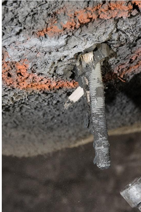
Figure 25. Bolt covered by hardened injection grout
