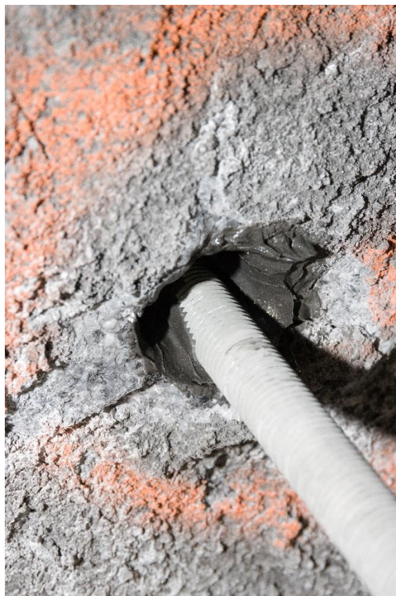
Figure 34. Void in outer part of bore hole.
