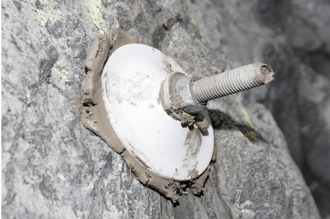
Figure 31. Successfully installed washer with puck on quite even surface,
