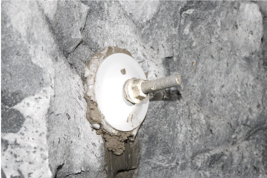
Figure 32. Installation with twin pucks: before installation (a) and after tightening (b).
