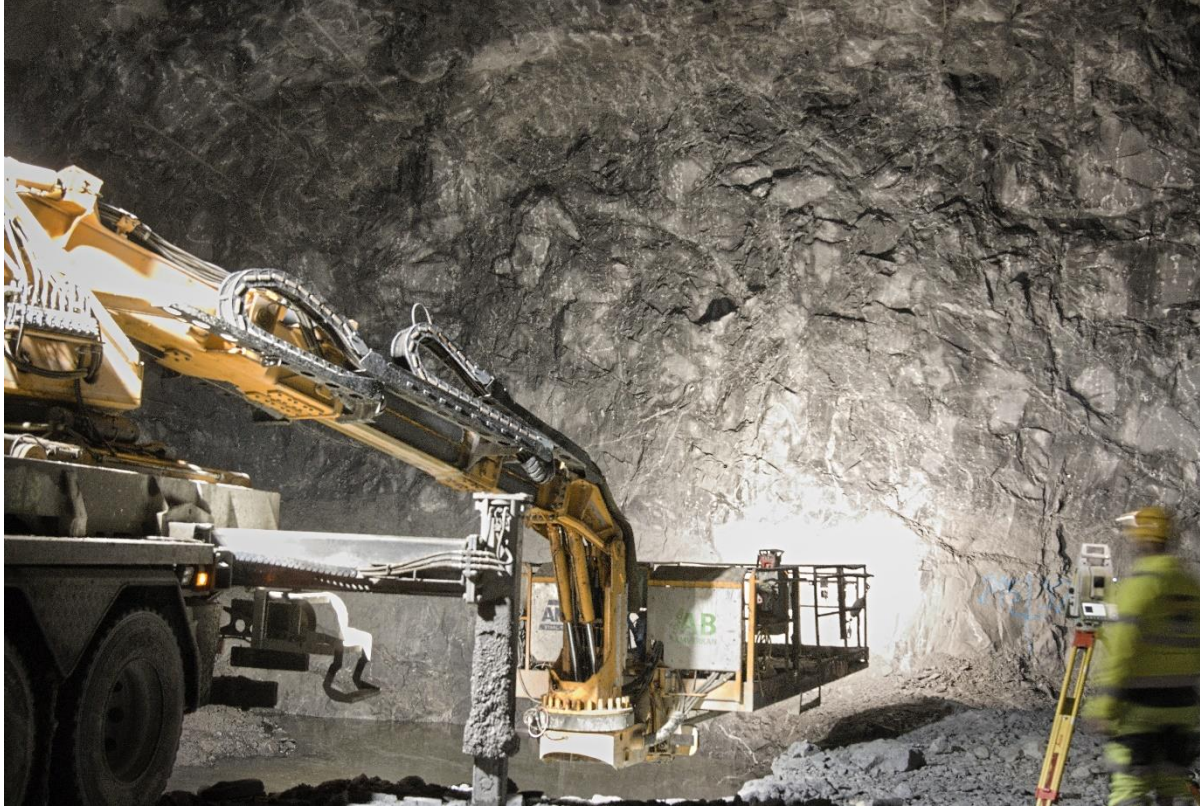
Figure 28. Working platform used for the tests.
