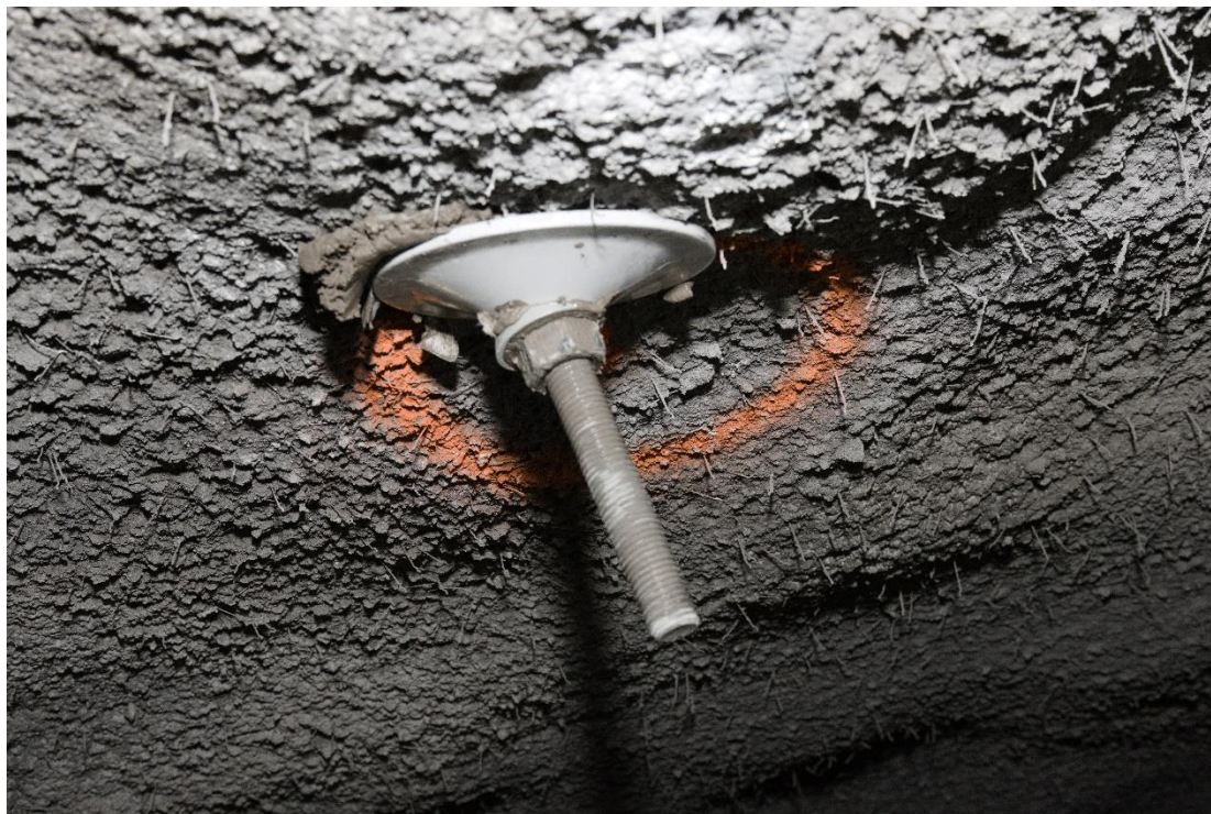
Figure 33. Installation in tunnel roof on pre sprayed rock.
