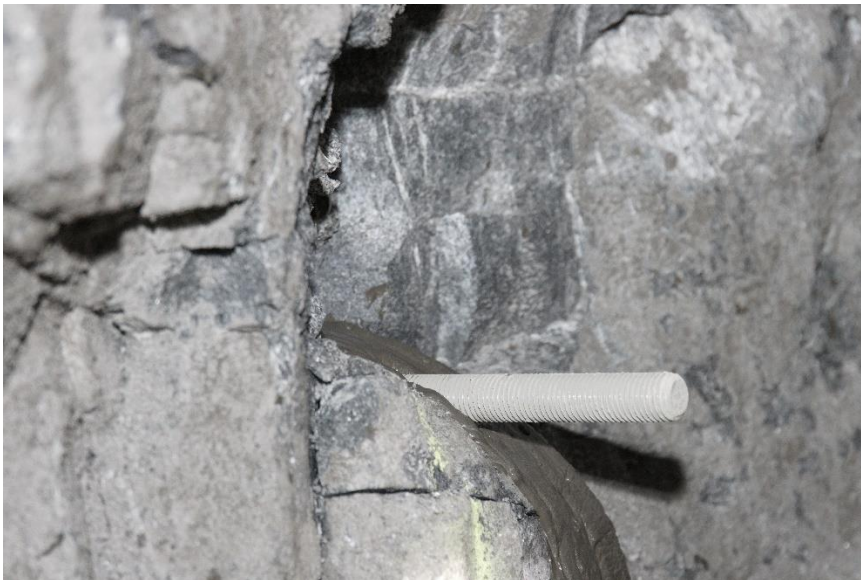
Figure 26. Bolt in the uneven rock surface with sharp corners
